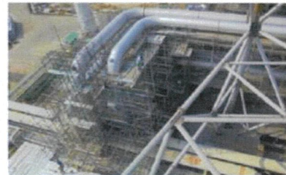
Tie-in 48" Flare Header OLE2-2 Complete
